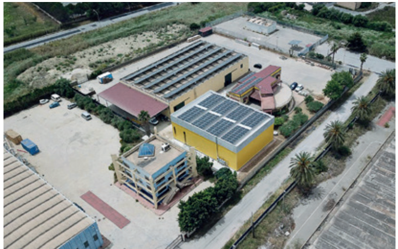
A job performed by the company
